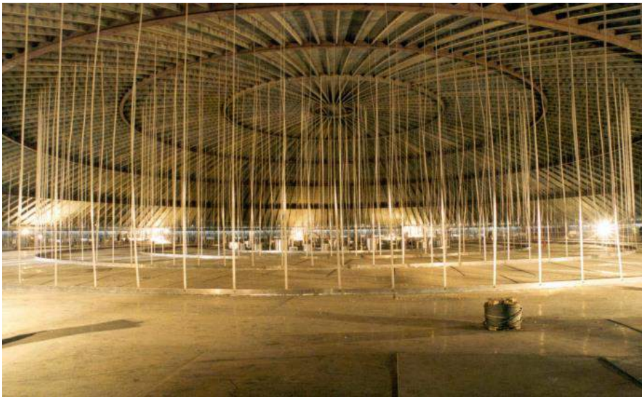
Figura 11. Interior tanque - Techo suspendido [10]
